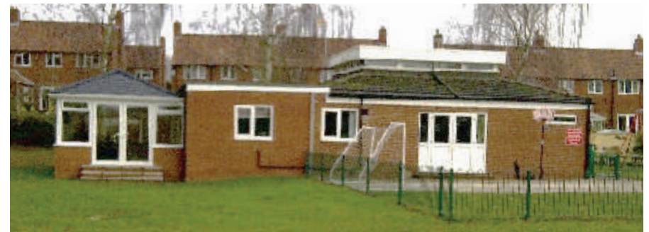
The Community Centre in 2014 with the Extension (2011) and Conservatory (2013)
